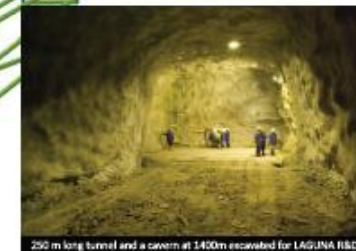
250 m long tunnel and a cavern at 1400m excavated for LAGUNA R&D
